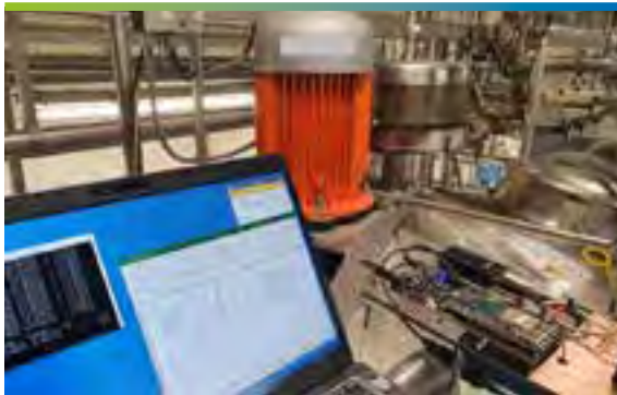
Testing of prototype Wifi system in a harsh factory environment
